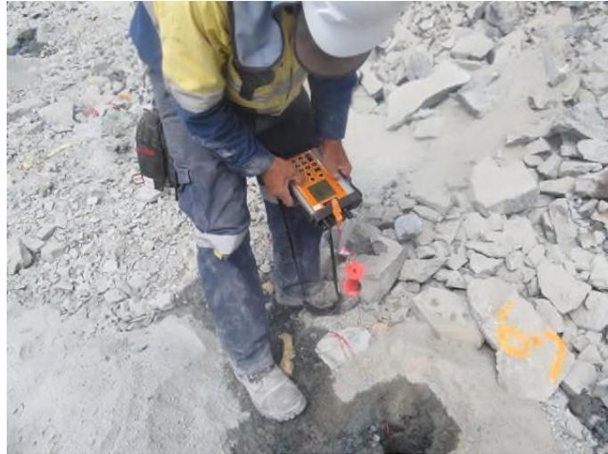
Figure 9 Logging of Electronic Detonator
